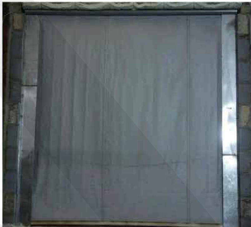
Fig. 8 Unexposed Side to Temperature/Time Resistance Test after 120 Minutes
