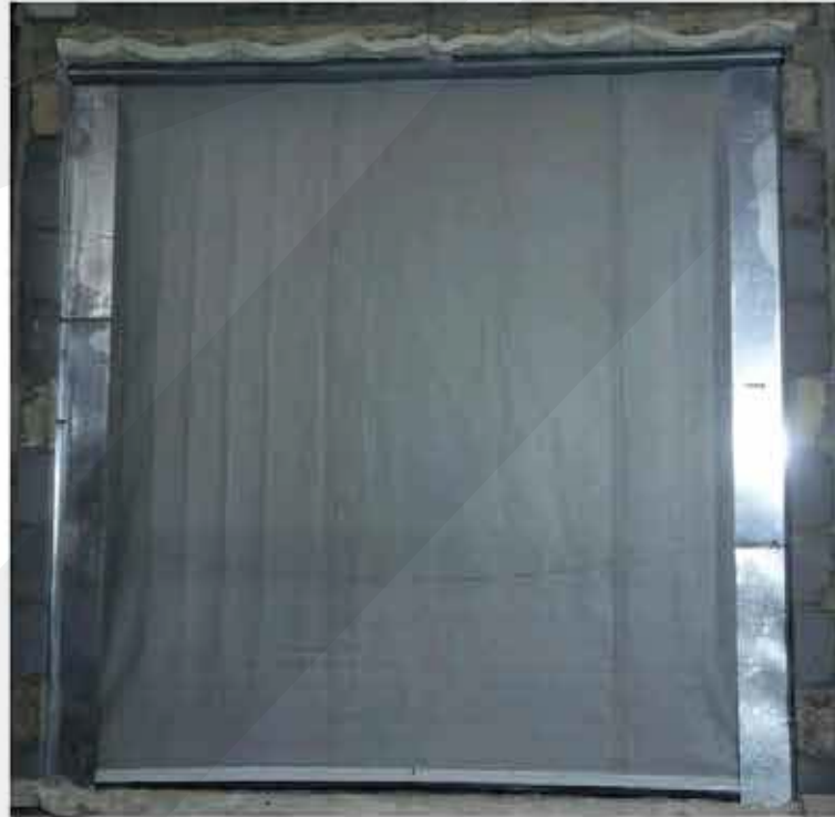
Fig. 5 Unexposed Side to Temperature/Time Resistance Test after 10 Minutes
