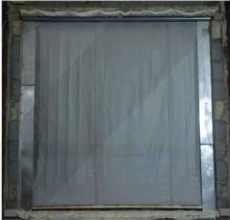
Fig. 7 Unexposed Side to Temperature/Time Resistance Test after 90 Minutes
